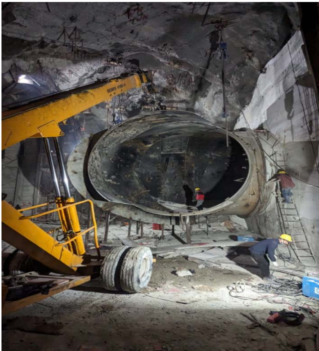
Bifurcation Lower Horizontal PS – 3.9 m dia. U/s of MIV
