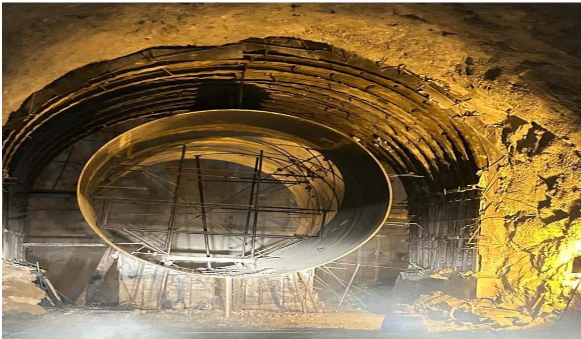
Erection of Steel Liners – PS 3
