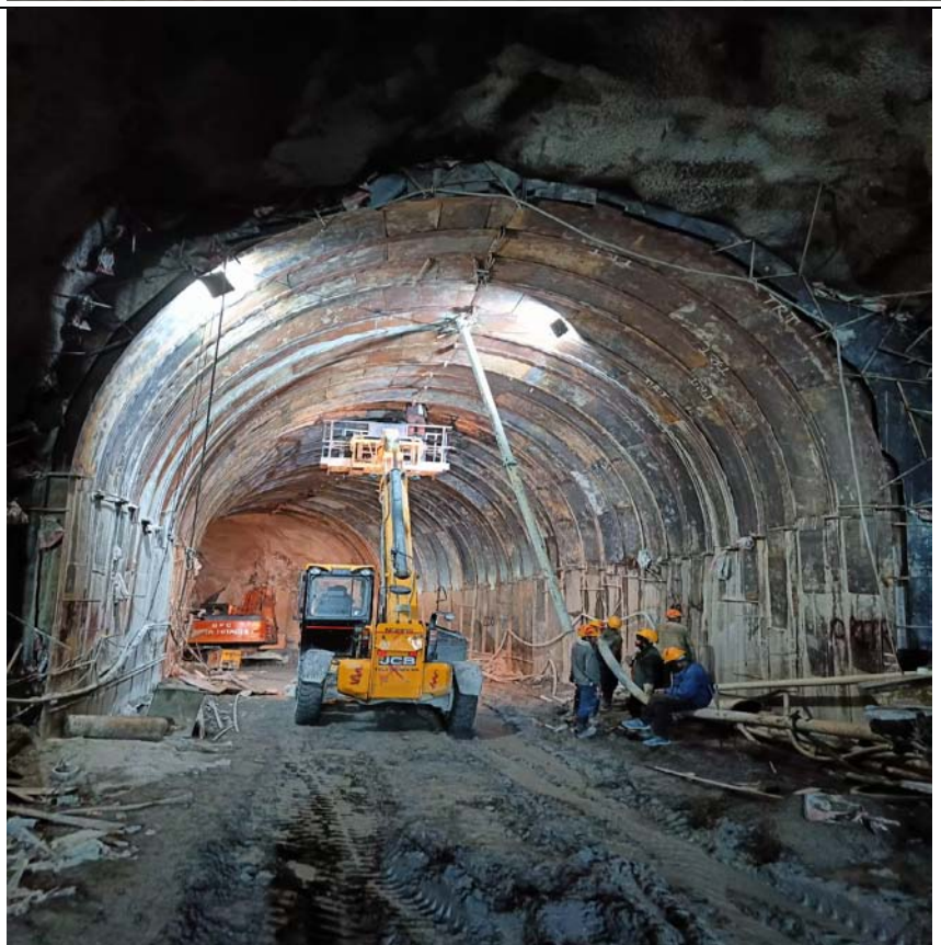
Adit to TRT
