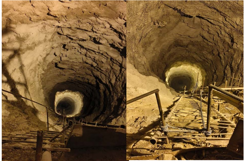
Inclined Pressure Shaft # 1
