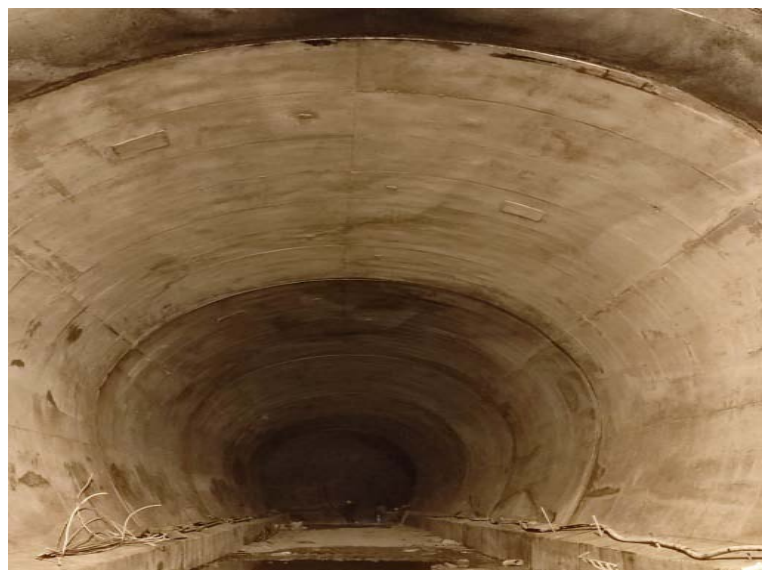
Concrete Lining of HRT
