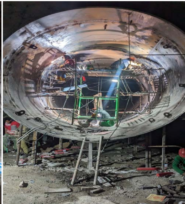
Bifurcation Lower Horizontal PS – 3.9 m dia. U/s of MIV
