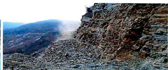
Dam Top Road
