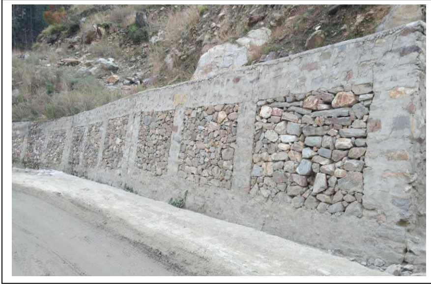
Protection Works at Pakal Dul Construction Sites to check Soil Erosion, Sliding etc.
