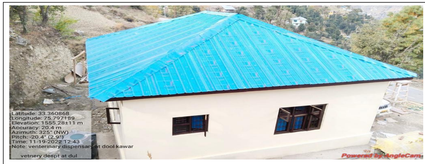
Construction of Veterinary Dispensary at Dool, Kishtwar.
