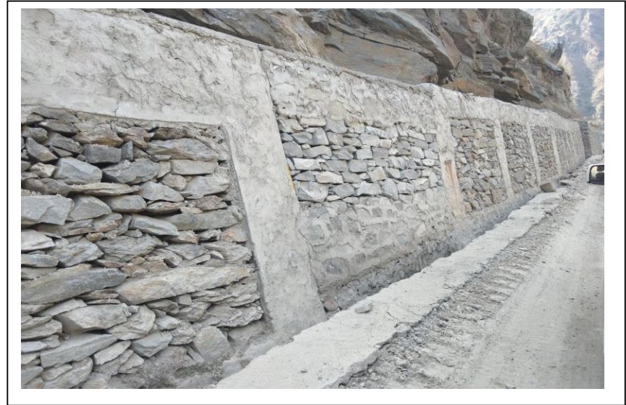
Protection Works at Pakal Dul Construction Sites to check Soil Erosion, Sliding etc.
